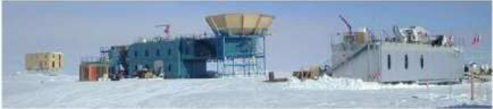
Figure 27: The South Pole Station. The AMANDA-II telescope electronics are located on the 2nd floor of MAPO, the blue building shown in this picture. [From http://www.amanda.uci.edu/ .]
