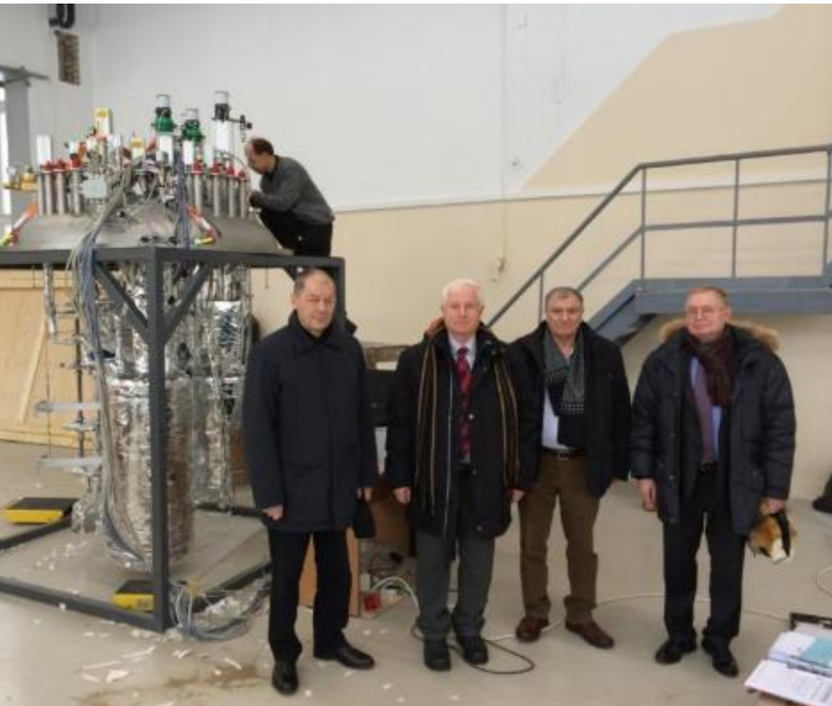
Satellite helium refrigerator during assembly on-site in October 2013.
