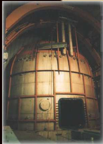
Borexino Water Tank with its big entrance door before the construction of the Big Building West and Clean Room
