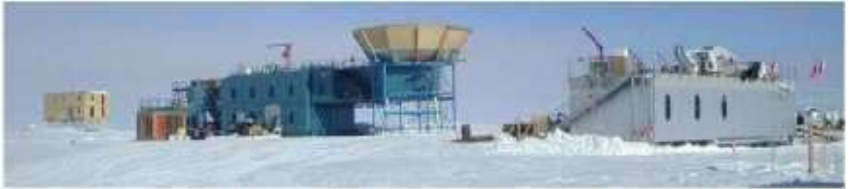
Figure 165: The South Pole Station. The AMANDA-II telescope electronics are located on the 2nd floor of MAPO, the blue building shown in this picture. [From http://www.amanda.uci.edu/ .]
