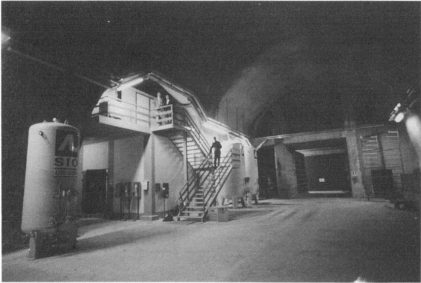
Figure 6.35. The experimental building of the Heidelberg–Moscow \beta\beta experiment constructed in the Gran Sasso underground laboratory by the Italian National Institute for Nuclear Physics (INFN). The lower stories house the detectors, the upper stories the computers and the data processing. A liquid nitrogen tank can be seen in the foreground. The large door in the background leads to Hall A, where LVD and GALLEX are located (see chapters 4 and 7) (from [Kla91f]).
