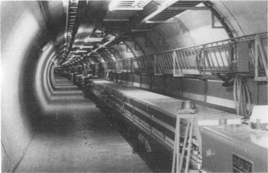
Figure 2.7. Top: aerial photograph of CERN. Geneva airport in the foreground, the French Jura in the background. In between are the LEP tunnel and (left) the SPS. The frontier between Switzerland and France is shown by dots (photo: Swissair). Bottom: view into the LEP tunnel, showing the pairs of dipole magnets (lighter) and the focusing quadrupole magnets. Note the low curvature of the tunnel (photo: CERN) (from [Scho89]).
